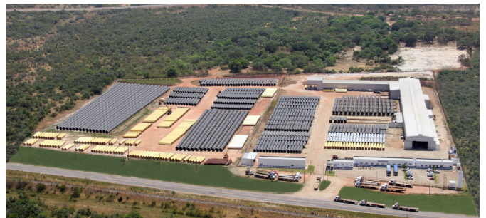
Plant in Caucaia – CE - Brazil (Steel pipes) Land – 320.000m 2 Construction – 7.471m 2
