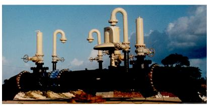
Operational safety in a water distribution pipes systems requires the control of elimination of the air accumulated on the top points during filling or air inlet in case of either desired or accidental pipe emptying.
