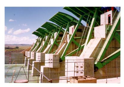
Tainter Gates are usually used to control the water level in a dam or water distribution channel. The Tainter Gates supplied by *hydrostec* are designed specially for a long working life under hard operating conditions.
